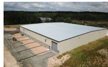
Example of shell building
